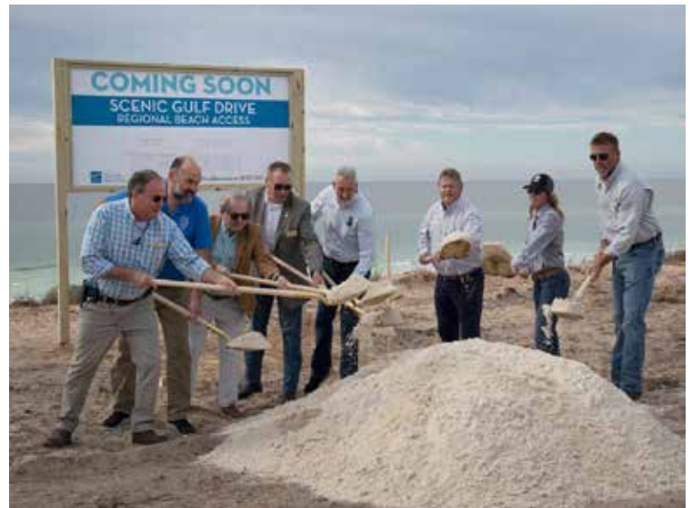
Representatives from the Walton County Board of County Commissioners and Visit South Walton break ground on the Scenic Gulf Drive Regional Beach Access.
