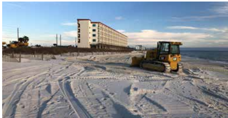
The Inlet Sand Bypassing Project is replenishing sand and enhancing the beautiful beaches of Mexico Beach.
