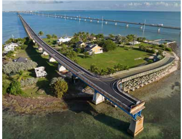
A scenic 2.2-mile section of the Old Seven Mile Bridge, serving as a linear park and gateway to tiny historic Pigeon Key, reopened in mid-January after extensive renovations.
